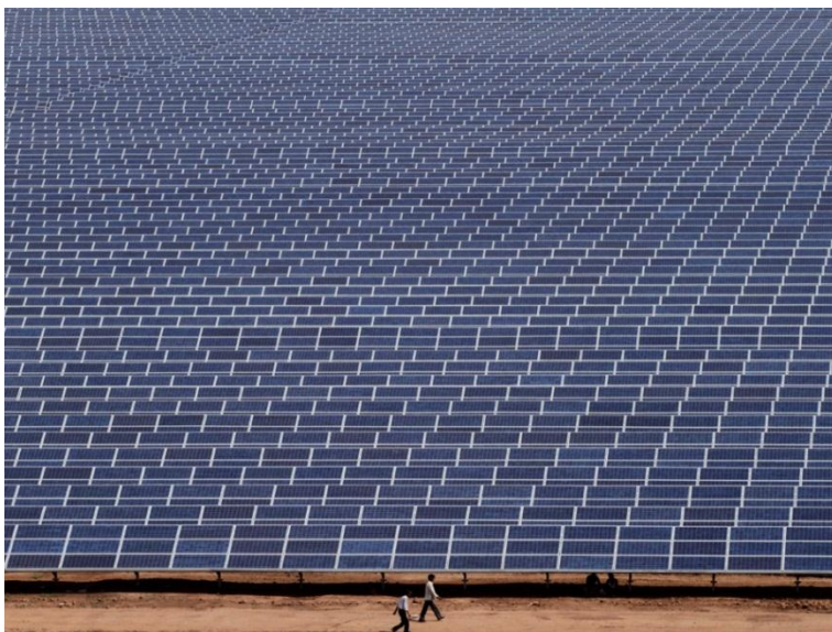
Picture 4: Gujarat Solar Park, India
