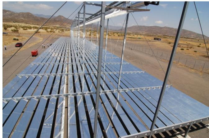
Picture 7 - Fresnel reflector in Almería, Spain
